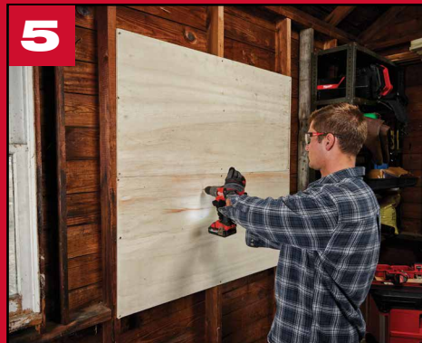
5 Pre-drill all mounting holes with a 3/32" bit.
