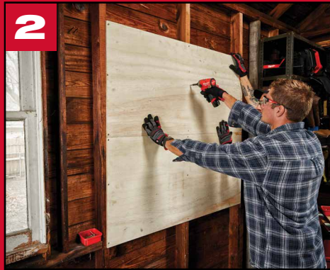
2 Attach plywood to studs with a minimum of 9 wood screws.
