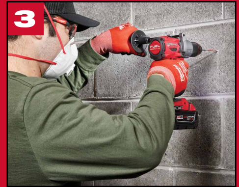
3 Pre-drill holes with 3/16" masonry bit.
