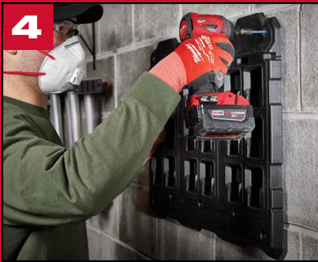
4 Using 1/4" x 1-1/4" concrete anchors, fasten the plate to the wall.
