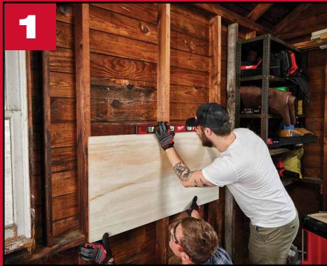
1 Have a partner hold up plywood backer in desired location and align it so it is in the center of a stud. Ensure plywood is level.
